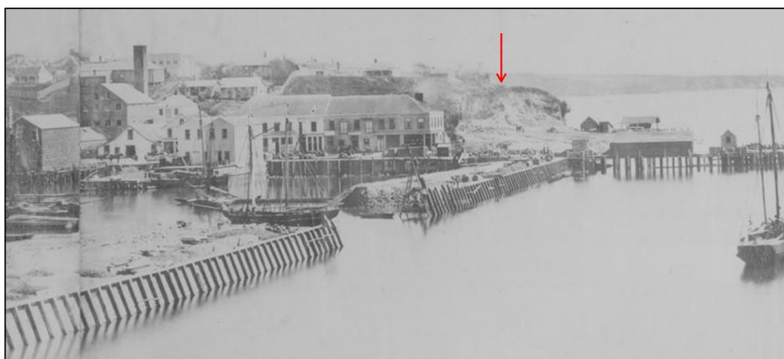
Figure 9. Photograph dated 4 October 1859, looking southwest from Point Britomart showing Commercial Bay during the early stages of reclamation, with Smale's Point under demolition (arrowed in red) (source: Auckland Libraries Heritage Collections, 4-1121)
