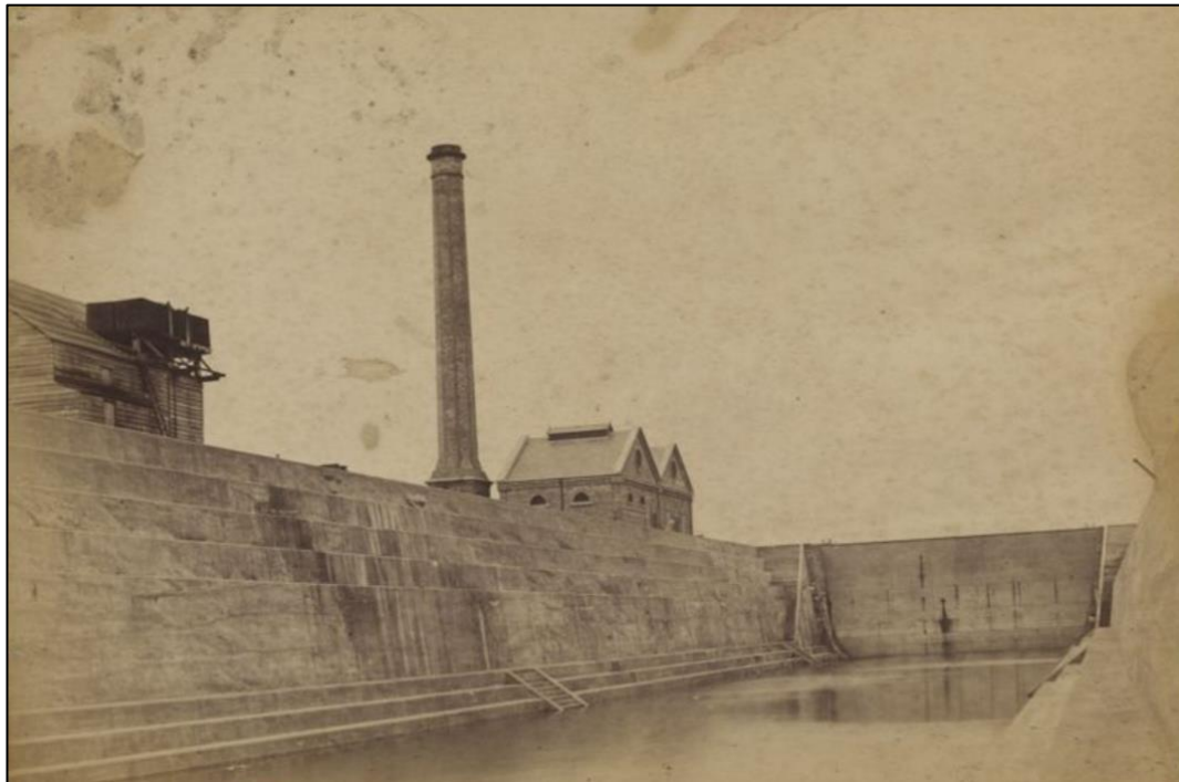
Figure 12. Photograph of the Auckland Graving Dock and engine and boiler house dating to the 1880s (source: Auckland Libraries Heritage Collections, 1677-056)
