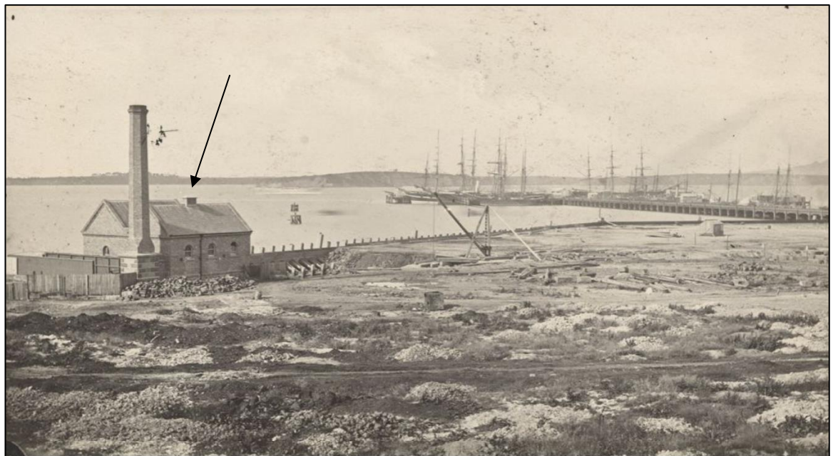
Figure 11. Photograph taken in the late 1870s from the foot of Hobson Street looking towards Queens Wharf, showing recently reclaimed land with the engine and boiler house of the Auckland Graving Dock indicated by arrow (source: Auckland Libraries Heritage Collections, 1043-122)
