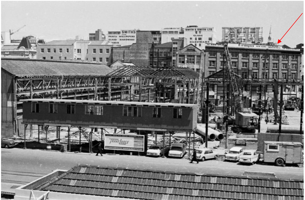
Figure 18. Photograph dated 1968 showing the demolition of the World War II warehouses as part of the construction of the Travelodge Hotel, with the Gunson Building visible in the background and indicated by red arrow (source: Auckland Libraries Heritage Collections, 786-A26-04)
